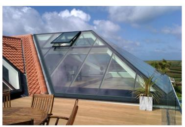
Working within the channel islands for a private client, the team a number of glazing provided element this substantially extended residential property. These glazed elements included: 2 triangular rooflights, hydraulically actuated access hatch onto the flat roof terrace, and the most impacting part of development was the main Dual Pitched Rooflight with a hipped end.
